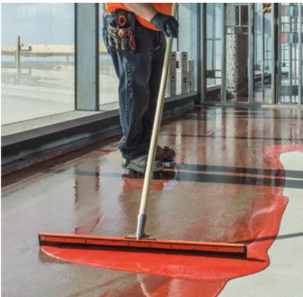
Like most hospitals, Jacobs Medical Center utilized a number of floor coverings for the service needs of diverse spaces. Prior to installation of vinyl sheet goods, all floors were prepared with a CustomTech<sup>®</sup> calcium aluminate cement underlayment system. The Rouse Company addressed floor flatness and moisture mitigation on 330,000 square feet of concrete slabs in the corridors, laboratory and patient care areas.
